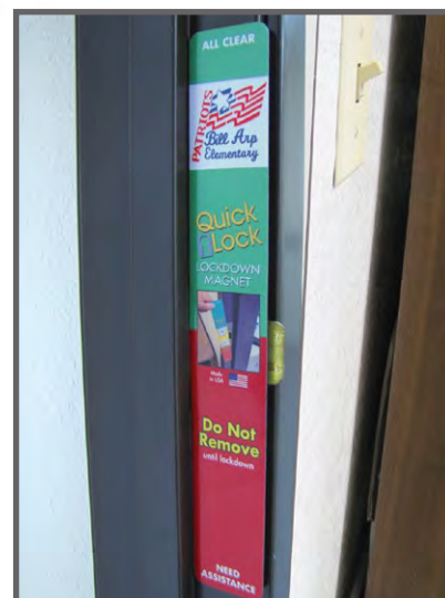
Magnet attracts to metal door jamb directly over latch plate. If lockdown occurs, remove magnet to allow door to lock.
